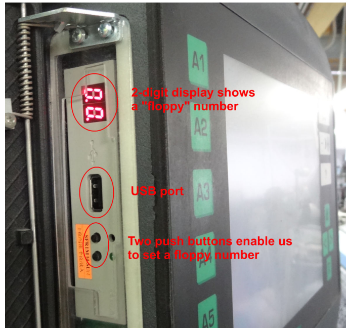
Figure 360: USB floppy emulator installed on Stäubli JC5 controller
